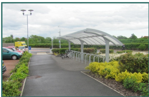
Cycle Stands and Shelter at Johnson Community Hospital
