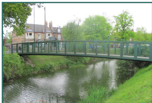
River Welland Footbridge
