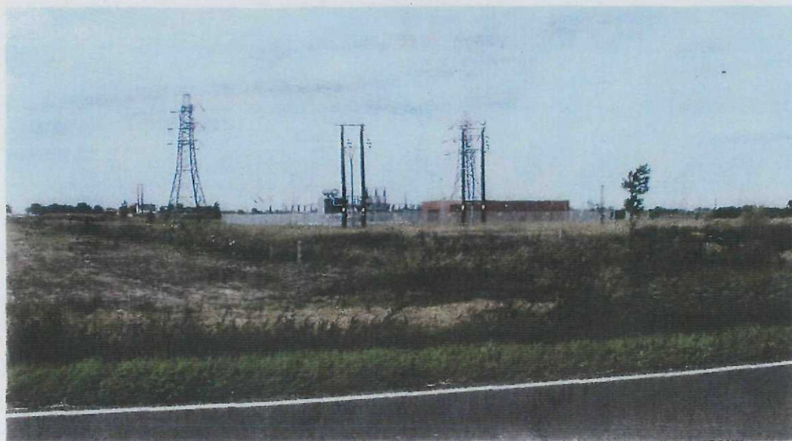
Power distribution infrastructure south of Holbeach
